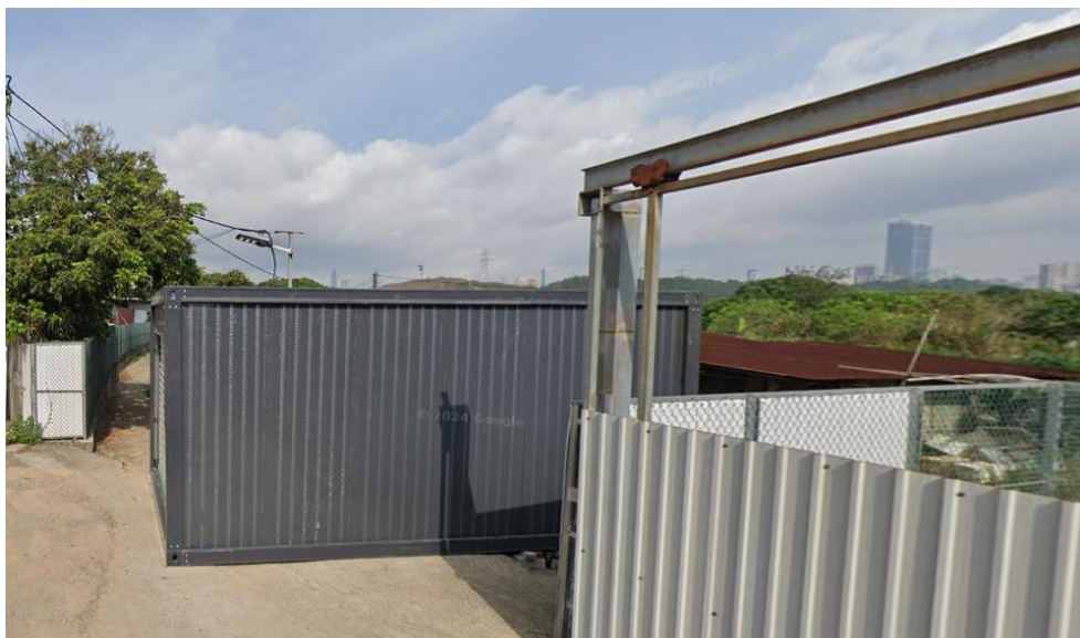
Figure 6. The East side of Lot Nos. 497, 498, 499 and 500 in D.D. 87
